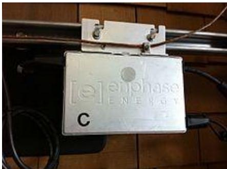
A solar micro-inverter in the process of being installed. The ground wire is attached to the lug and the panel's DC connections are attached to the cables on the lower right. The AC parallel trunk cable runs at the top (just visible).
